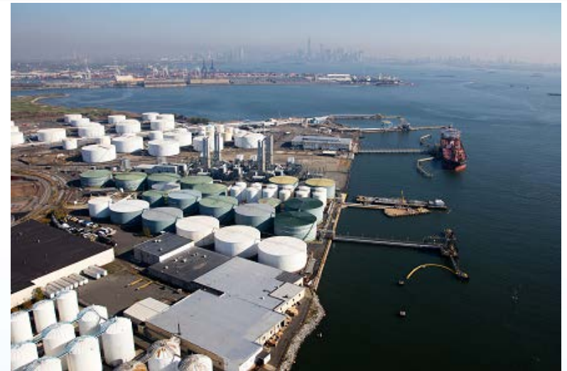
Buckeye Bayonne Terminal
