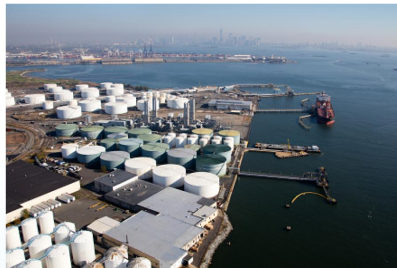
Buckeye Bayonne Terminal
